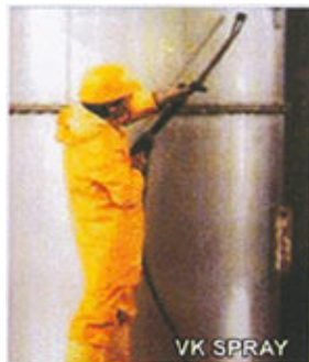
External application of VK Spray with special pressurized plastic spray bottle
